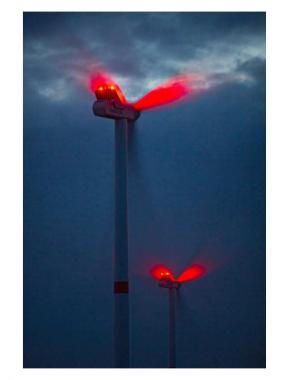
Need-based obstruction lighting means that the identification will only be activated if a flying object enters the airspace.
